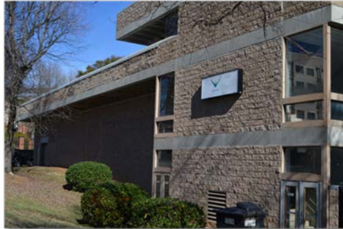
Atlanta Workplace Development Agency building
