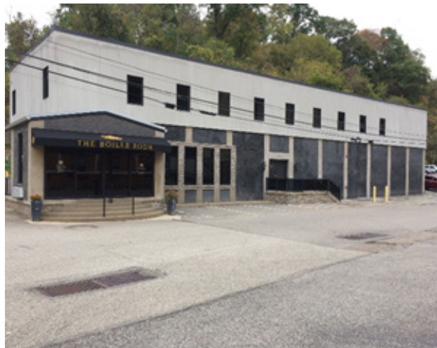
Location where Ventrone kept expensive equipment he purchased with Boilermaker funds
